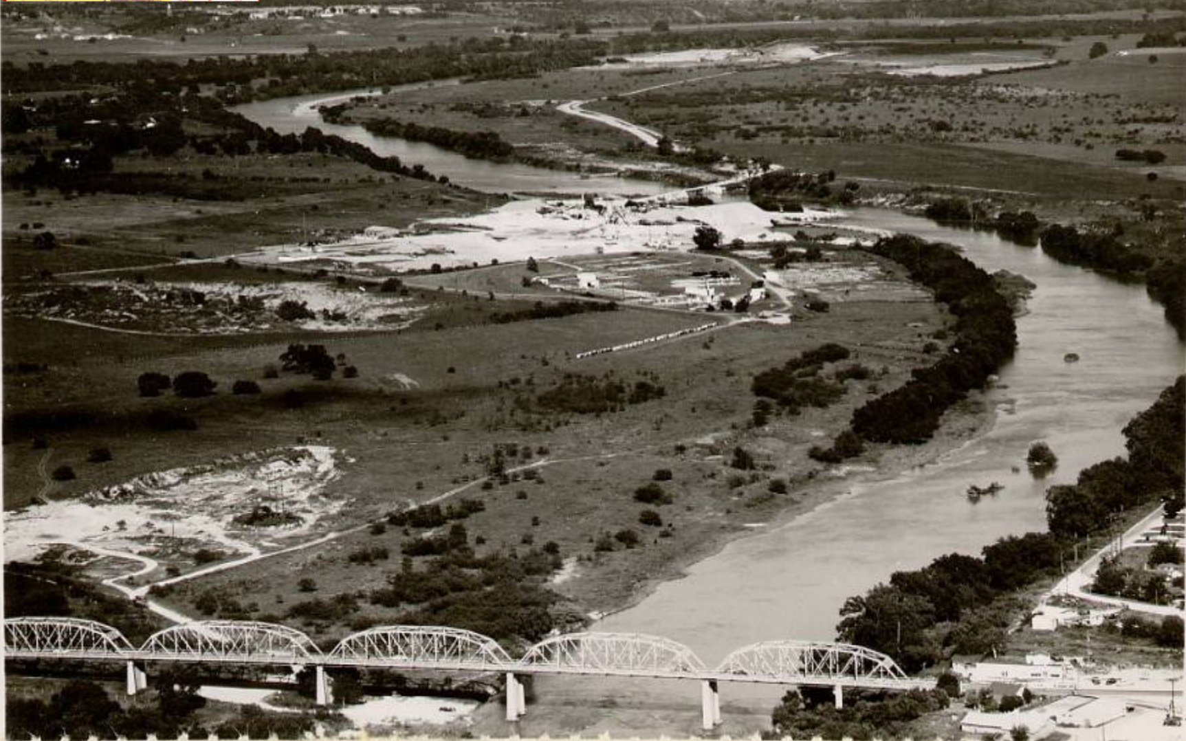
3402 Montopolis Bridge, Colorado River, south of Austin
